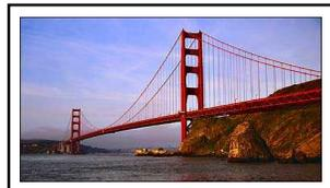
**SUSPENSION BRIDGE:** A suspension bridge works by hanging (suspending) the Deck of the bridge from flexible chains or ropes. The simplest form is made from wood and rope. The bridge can span from 2,000 to 7,000 feet – farther than any other type of bridge! Most suspension bridges have a truss system beneath the roadway to resist bending and twisting.
