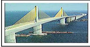
**CABLE STAY BRIDGE:** Newer than the other types of bridge. Large upright steel supports are used to transmit the load into the ground. Strong steel cables are stretched between the supports and the deck. This gives a distinct appearance to the bridges.
