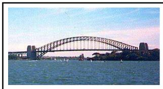
**ARCH BRIDGE:** Probably the oldest of its kind has a great natural strength. Romans built arches of stone. Today most arches are made of steel or concrete, and they can span up to 800 feet.
