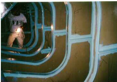
Fig 2. Ballast Tank showing multiple bays maintenance burdens for ship owners
